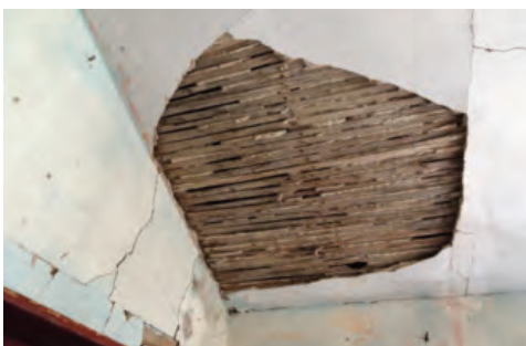
Lath and plaster ceiling exposed at the inn.
