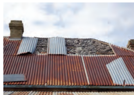
Shingles beneath the iron roof.
