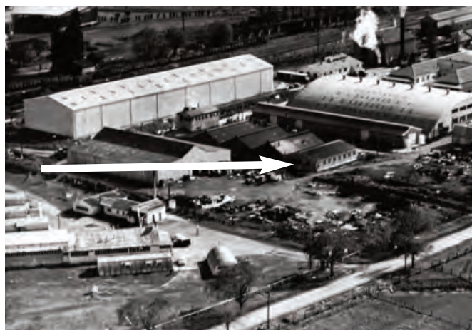
The location of the foundry towards the southern end of the factory site.
