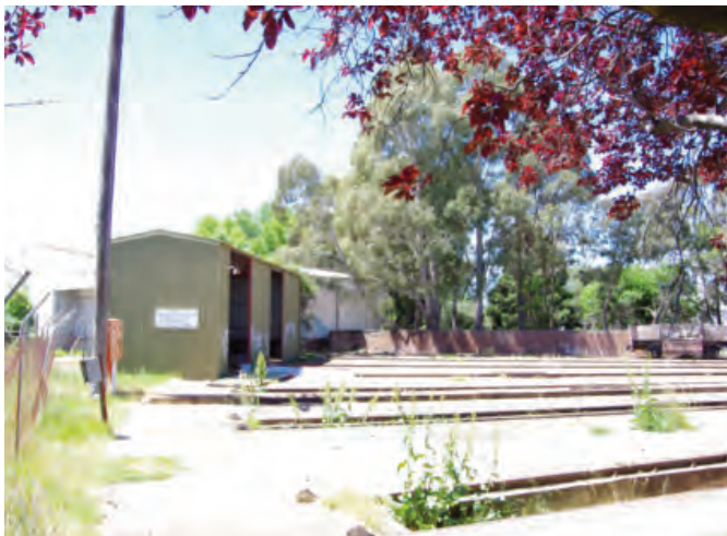
The shed erected by The Central West Railway with grant funding in 991-92. Occupation of the site was granted by the then State Rail Authority. Photo; Euan Greer, 29.10.2014.
