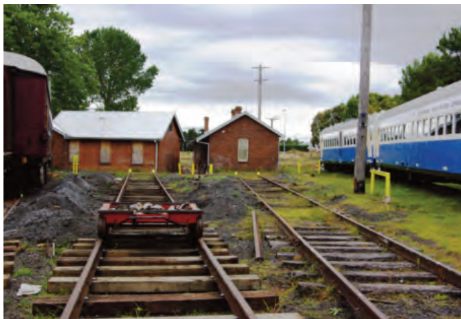
An example of the trackwork to be done throughout the depot. Photo; Euan Greer, 2.03.2022.
